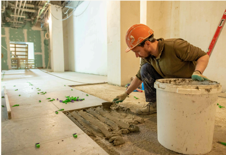
Tiling & Marble Installation
