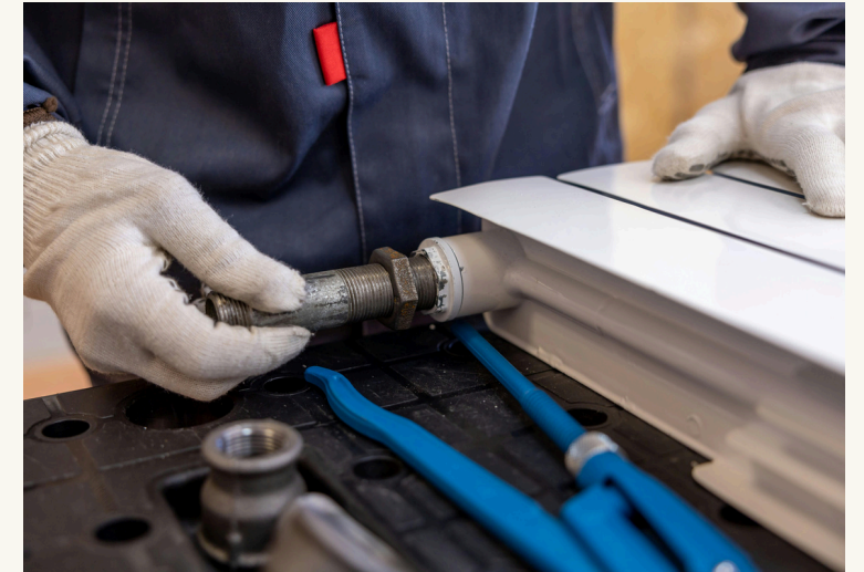
Plumbing & Piping Works
